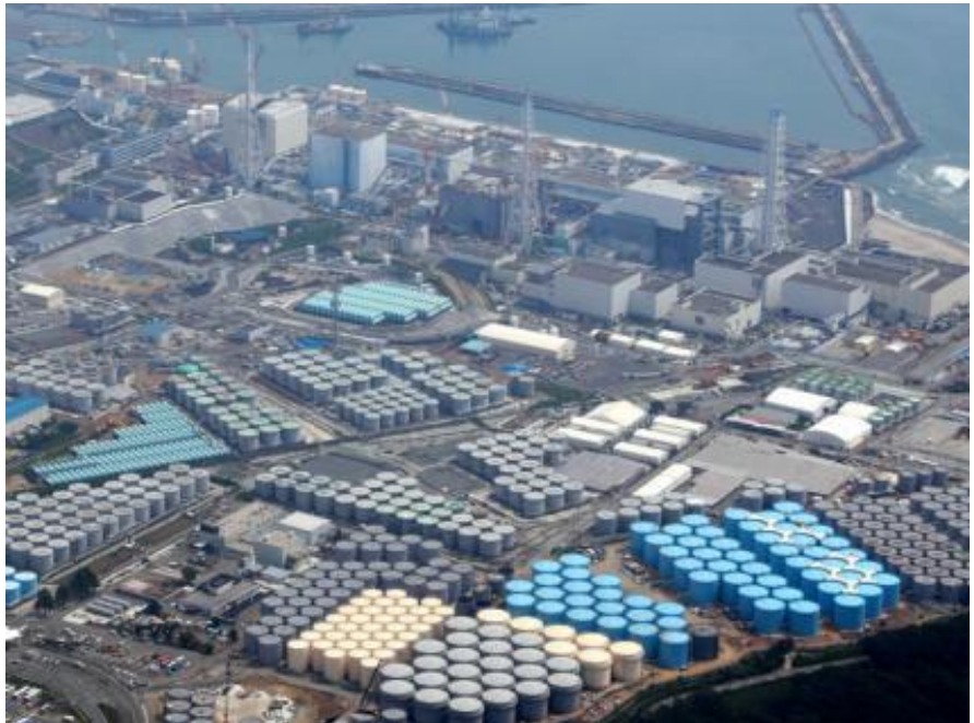
Wastewater storage tanks at Fukushima Daiichi NPP
